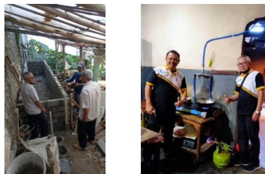
FIGURE 8. Biogas plant construction in household scale
