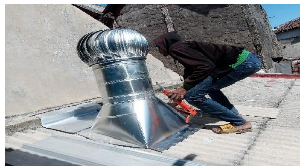
FIGURE 1. Installation in Patient 1's home
